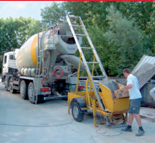
Einfache Stahlfaserzugabe in den Fahrmischer. Steel fibres can be easily added to the cement mixer.
